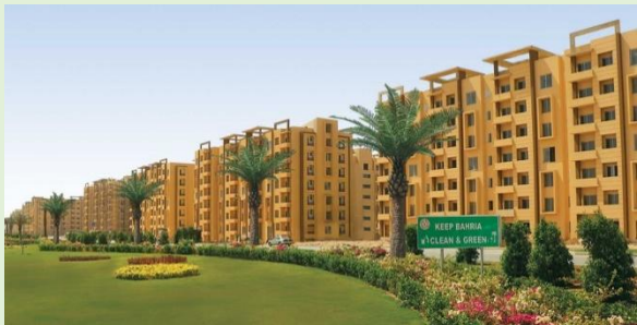
Multi-Story Structure (Residential + Economic) 33,065
